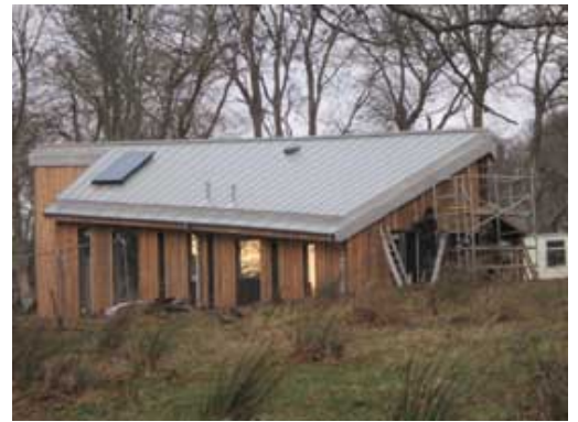
The Studio - almost finished
